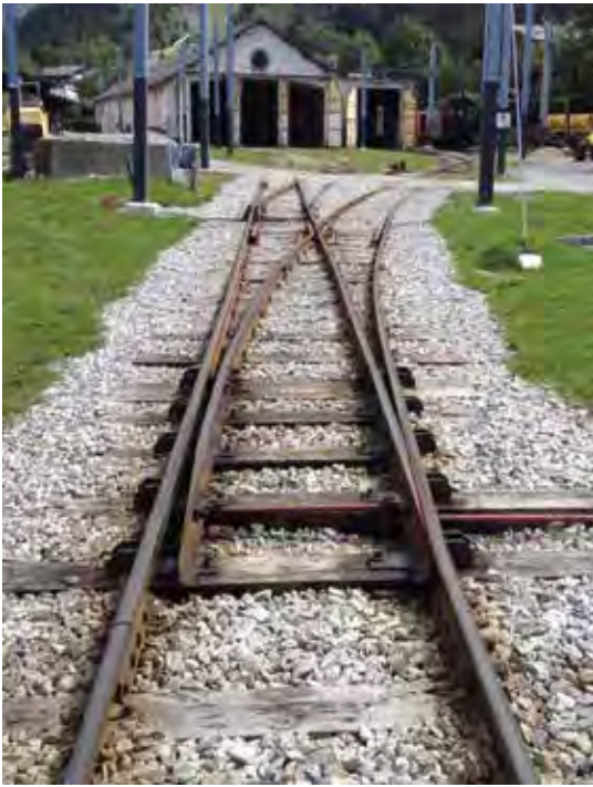
Aiguillages - écartement = 1000 mm Switches - gauge = 1000 mm
