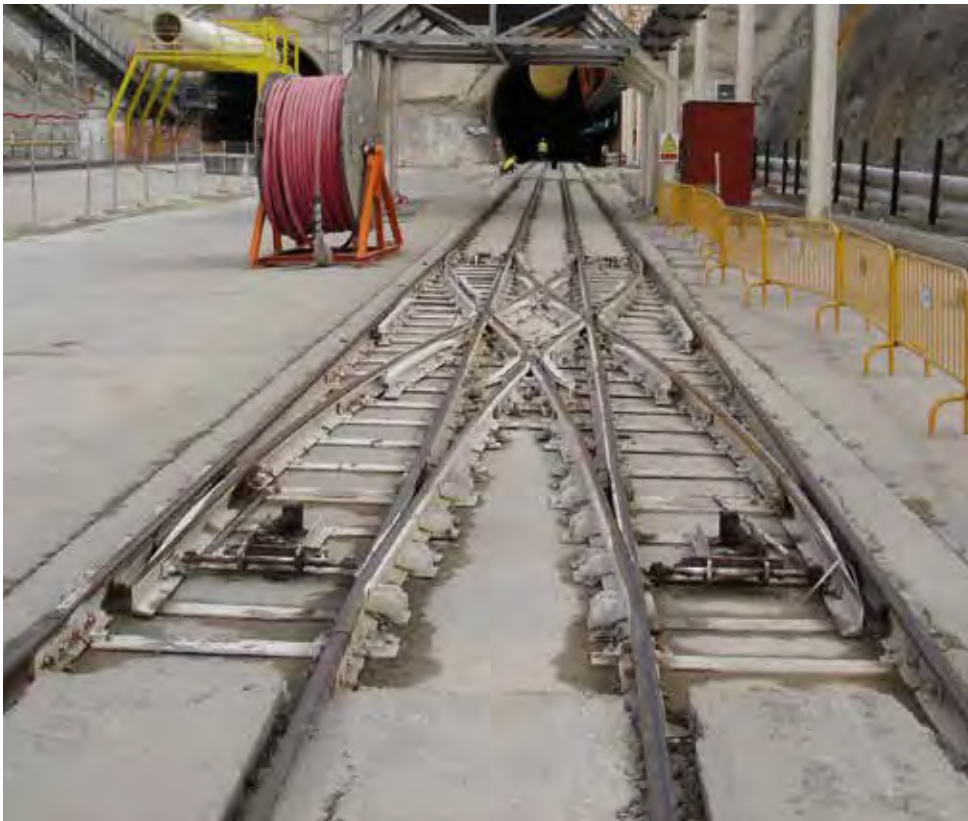
Communication double Double cross-over
